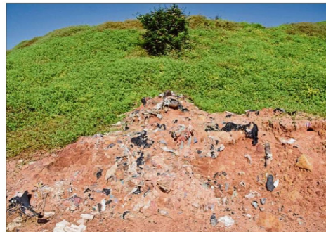
Mountains of muck remain piled up, camouflaged by a thick overgrowth.
