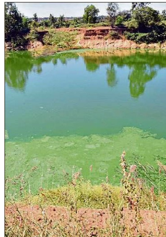
This leachate escape pond at the Mandur landfill site is filled to the brim with rainwater and leachate. The contaminated water percolates into the groundwater.
